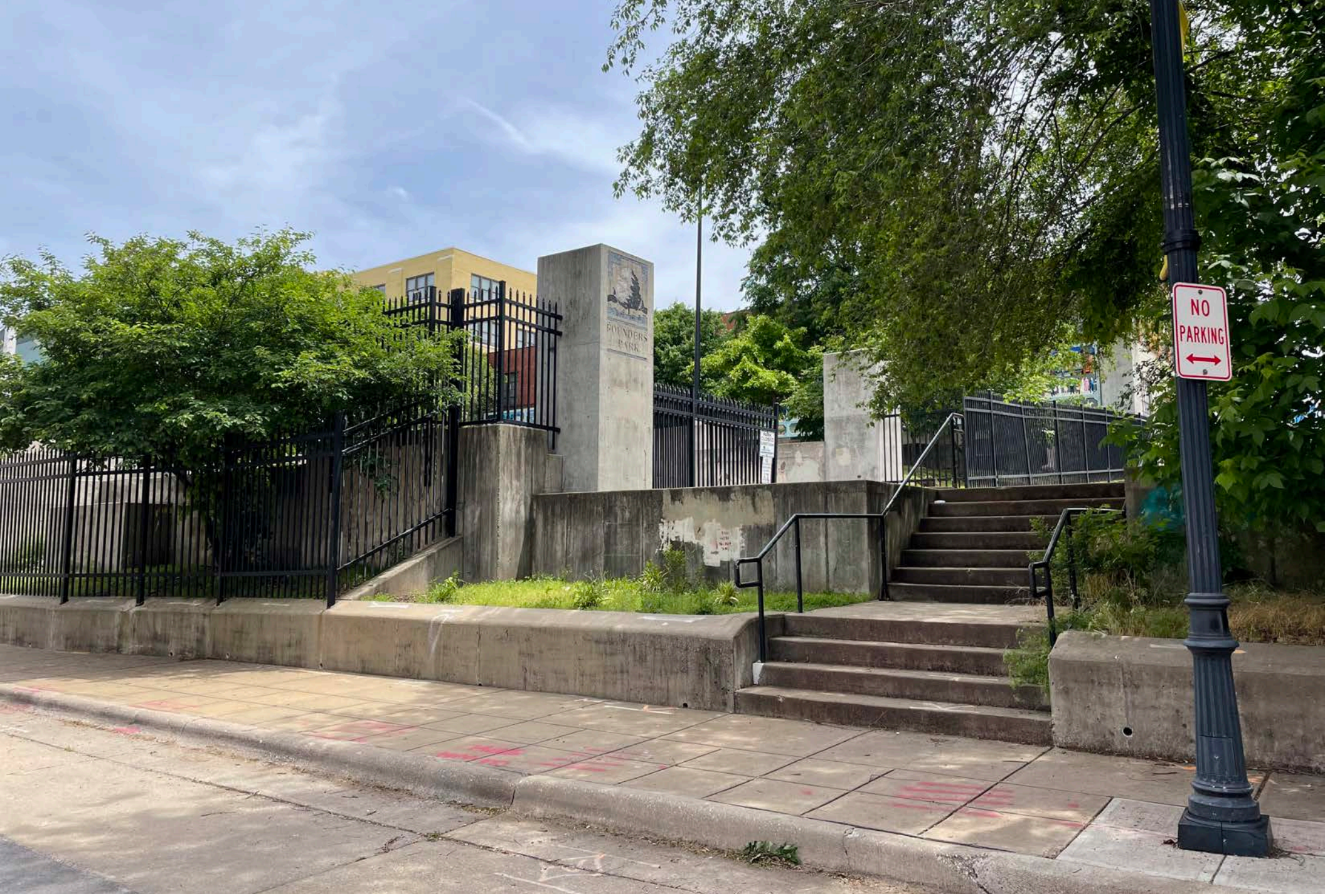
Figure A.7 North Robertson Avenue and East Water Street looking southeast
