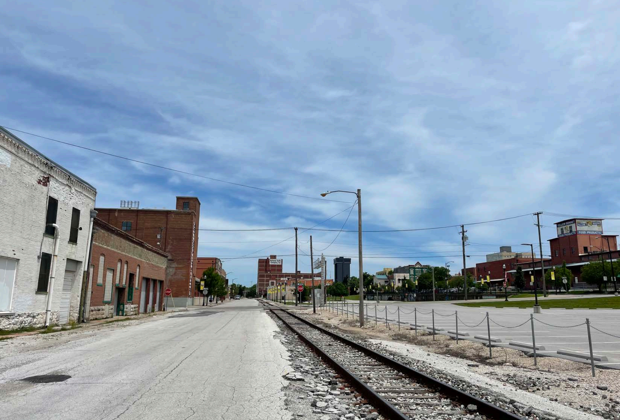
Figure A.4 West Mill Street looking east
