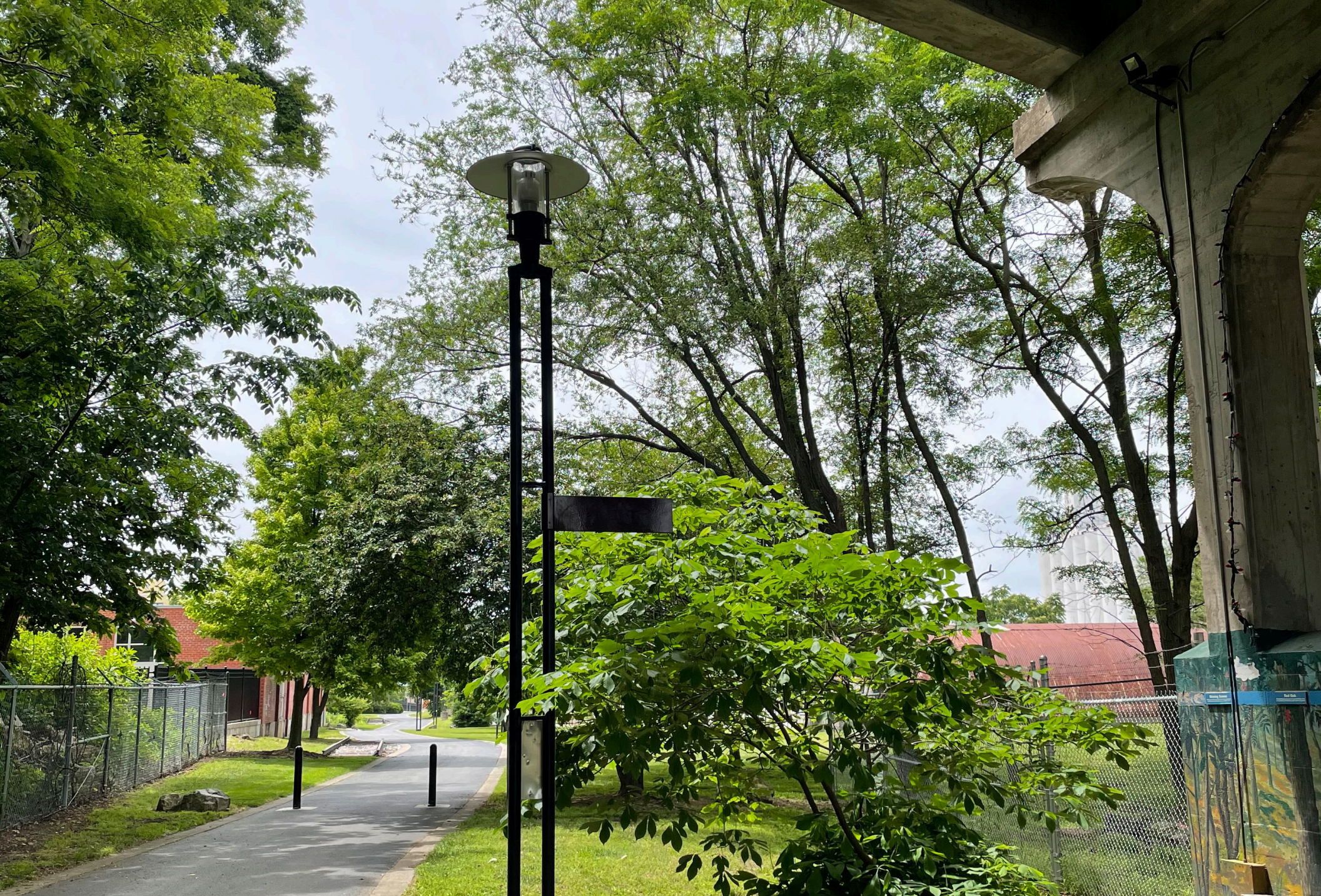
Figure 2.3 Jordan Valley Greenway underneath North Benton Avenue Bridge
